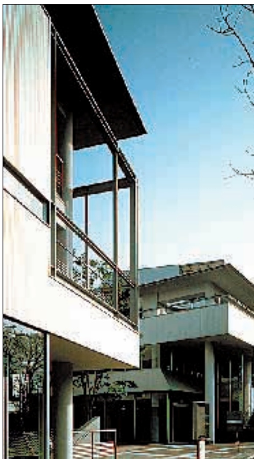
Inside job: Hillside Terrace phase VI
